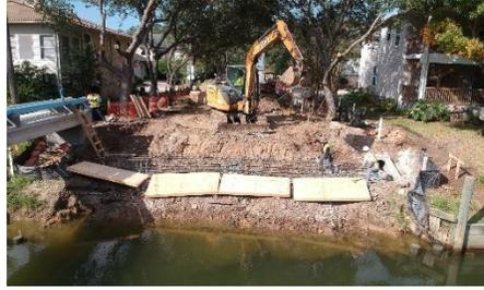
*Birch Road Bridge – Construction of bridge abutment*
