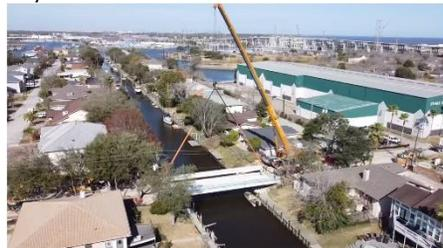
*Birch Road Bridge - Installation of Bridge Beams*
